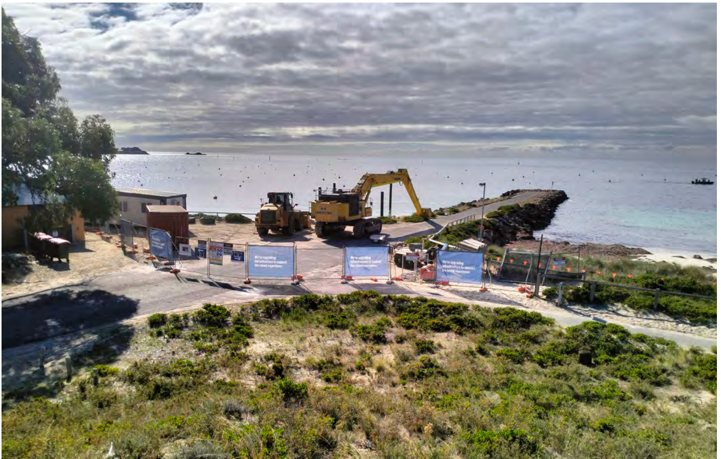
Preparations begin for new Barge landing area
